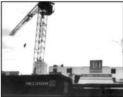
Building a condominium
